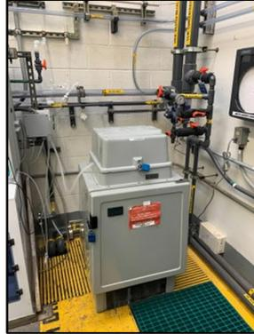
**IWD-5: pH Neutralization tank of the CH6 AWN System (Metal Finishing Compliance Point for CH6 facility)**
