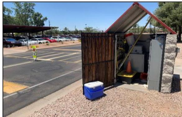
**IWD-8: Sampling valve on Discharge piping following last stage of cyanide treatment system located northwest of UPW Water Purification System (Metal Finishing Cyanide Compliance Point for CH1 facility)**
