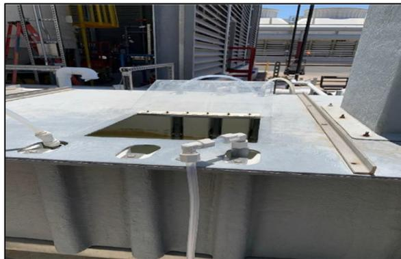
**IWD-10: Sampling valve on the Discharge side of the RGC tank prior to entering the CH8 AWN treatment system (Metal Finishing Cyanide Compliance Point for CH8 facility)**
