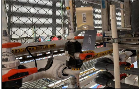
**IWD-9: Sampling connection in AWN weir after the CH8 AWN treatment system (Metal Finishing Compliance Point for CH8 facility)**
